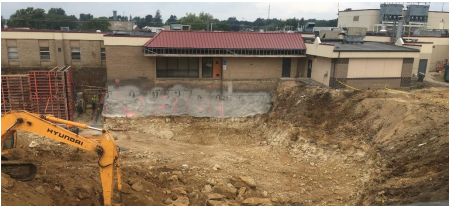
The excavation where Monroe Street used to sit is expanding to encompass the footings and foundation for the new Clinic and Med Surge addition.
