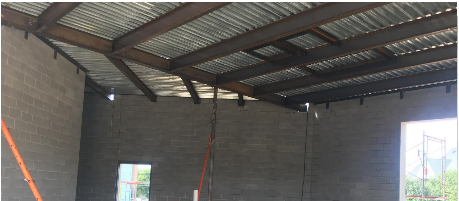
Another view of the Ambulance Garage. Here the block is complete and the steel structure and decking has been set into place.
