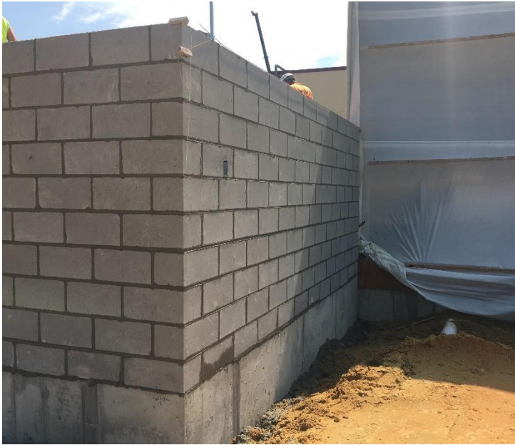
The Ambulance Garage walls being built where the garage will connect to the new Emergency Department.
