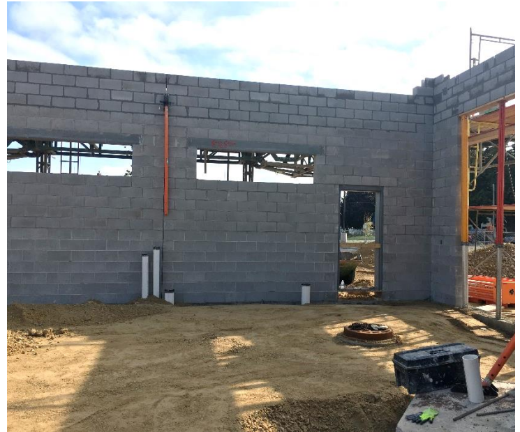
Almost-finished walls of the Ambulance Garage outline where the doors and windows will be located.
