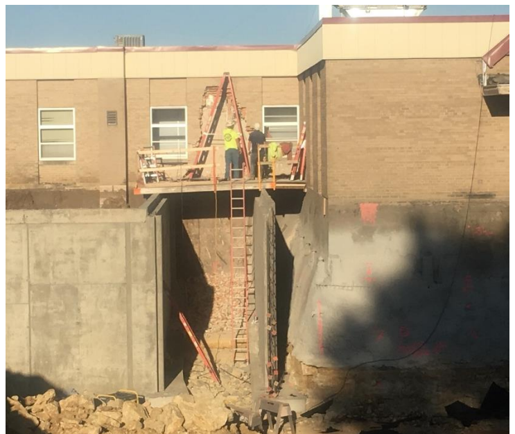
The crew here is working together to break through into the existing building to place two new columns and beams.
