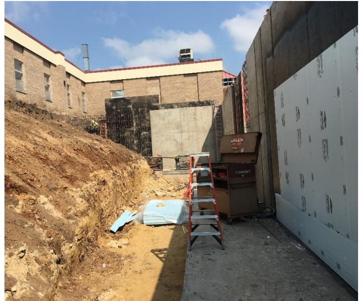
This is a view from the existing building side of the new walls. The walls are sprayed with a waterproofing coating and lined with a foam insulation.
