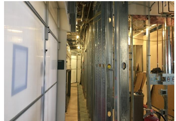
Three new exam rooms shown to the right of the Edge Guard barrier system that is visible throughout GRHC.
