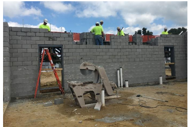
The masons are working hard to finish the block for the new Ambulance Garage.
