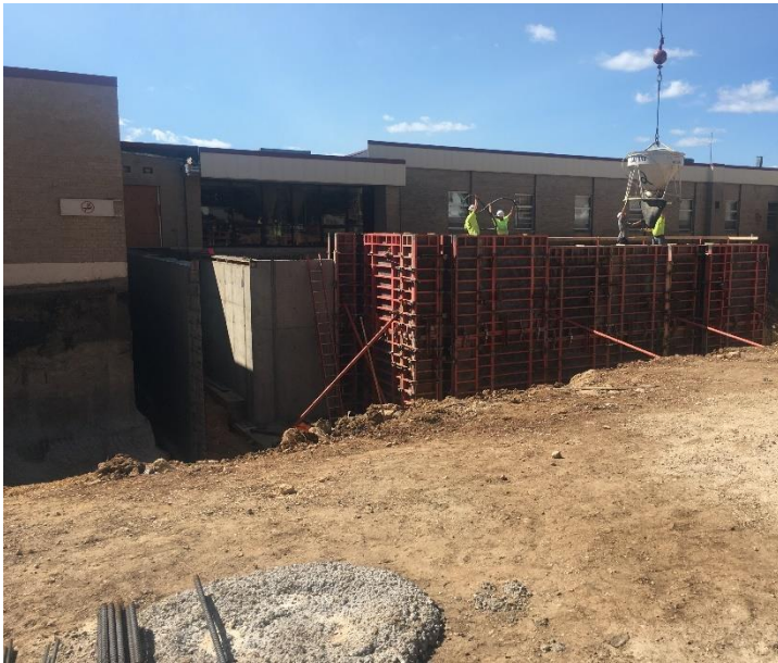
These tall walls act as a retaining wall and a foundation wall for the new Clinic and Med Surge addition.
