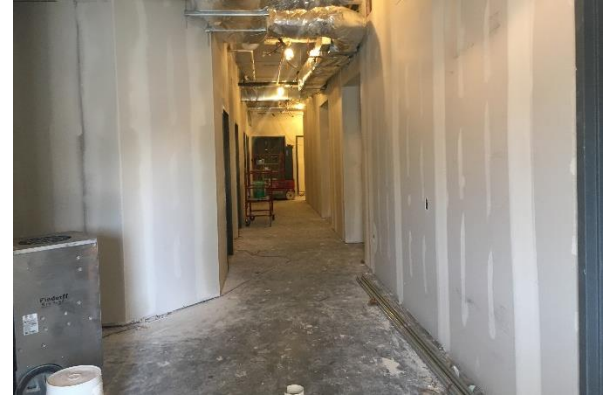
The new Education Area has walls, and will soon have a floor and other finishes as well.
