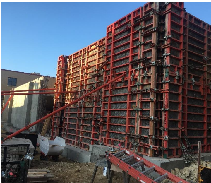
A closer view of the formwork used to build the footings and foundations. The team uses Peri formwork panels.
